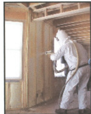
Soy insulation is available as a spray-on foam, as well as in panels.
